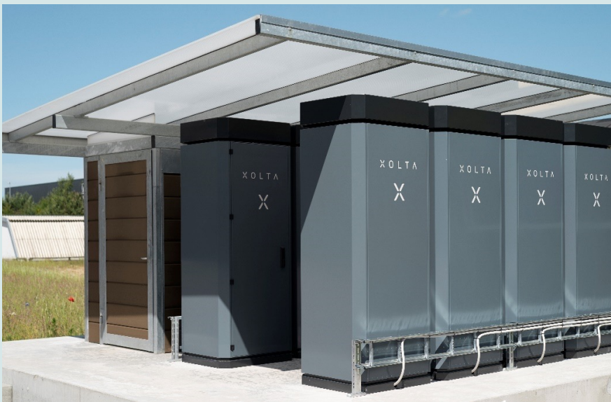
Figure 12: Haarup's machinery factory at Silkeborg has installed 12 XOLTA batteries that store electricity from the factory's solar cells and make the factory self-sufficient with electricity from March to November [22].
