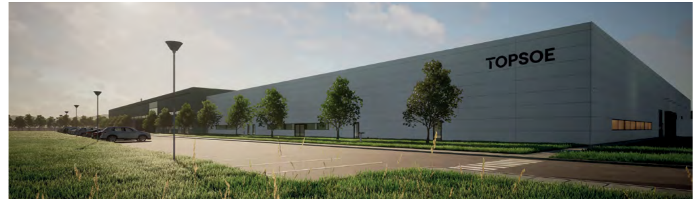
Figure 19: Visualisation of Topsoe's SOEC production plant, designed to produce SOEC annually equivalent to 500 MW electrolysis from expected 2025 with options to expand to 5 GW.
